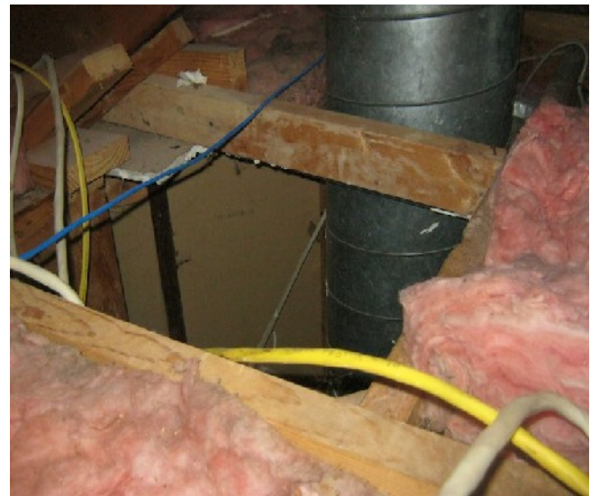
Visible Light Images of Thermal Bypasses
